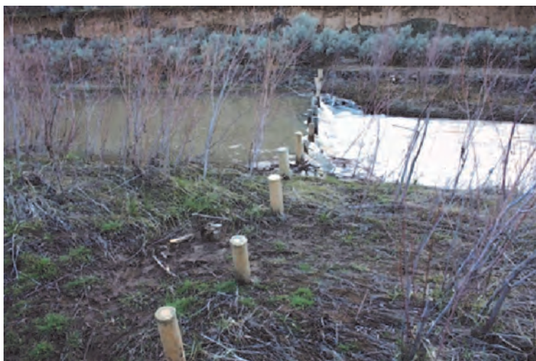
Figure 53. An example of a beaver dam support structure (BDSS) used in the Bridge Creek IMW to encourage beaver to build dams on stable structures. Dams are expected to entrain substrate, aggrade the bottom, and reconnect the stream to the floodplain.
