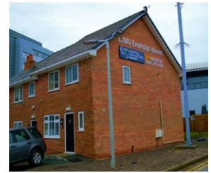
Figure 2. 2010 BRE Exemplar Houses used for testing at Liverpool John Moores University
