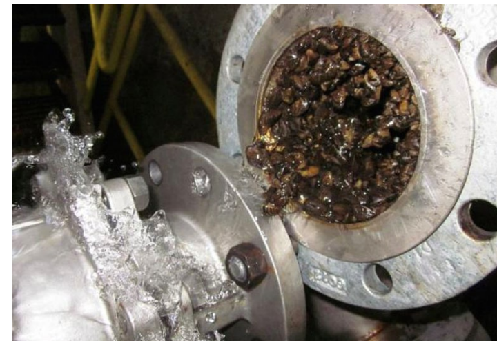
Dense colonies of zebra mussels can clog intake pipes. 📷 : Marrone Bio Innovations
