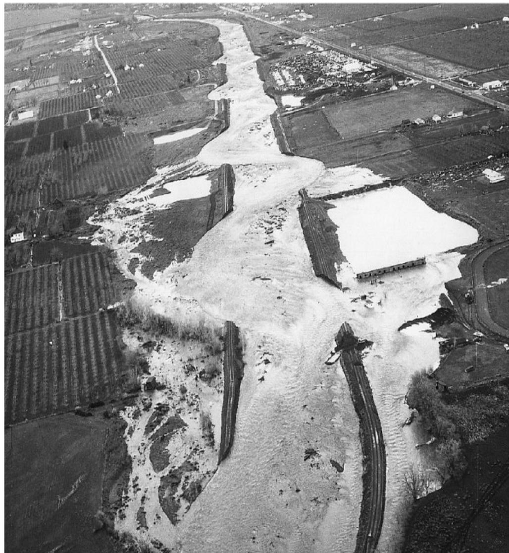
Figure 11.—Walla Walla River in the 1964 flood showing meanders in a channelized section near Milton-Freewater. (Source: OSU Archives)
